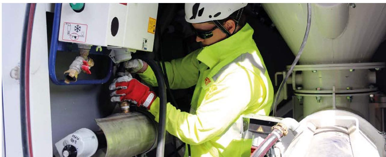
Connect the water supply hose to the water heater.
