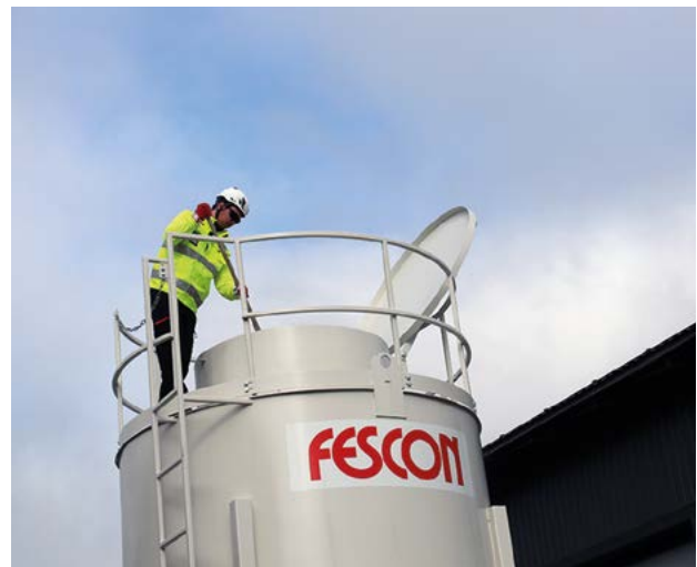
After loading the silo, the lid of the loading hatch must be carefully cleaned and closed.
