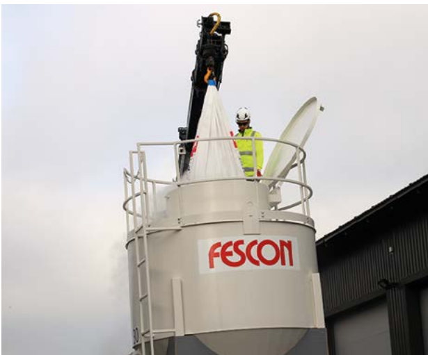
For deliveries arranged by Fescon Oy, the recipient must assist in the loading of the silo at the worksite by climbing on top of the silo.
